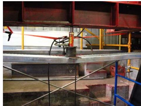
Point load failure at 1,850 lbs.
